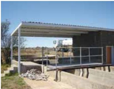
New installed walkway over grit channels to ease the cleaning of the screens.
