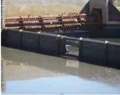
One of four horizontal shaft aerators that will be replaced with internal pasveer ditch wall to be repaired
