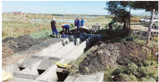
Cleaning of inlet works at the WWTW
