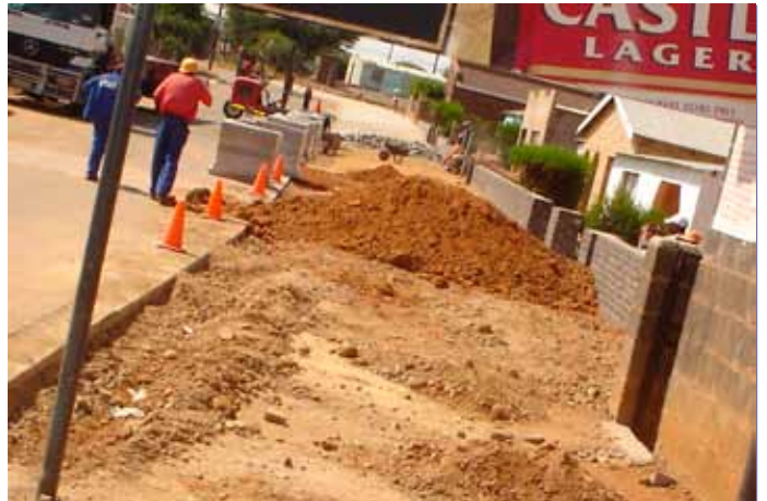
Preparing pavement for the laying of paving
